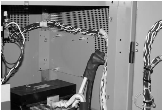
**Figure 2 - bracket mounted in unit**
